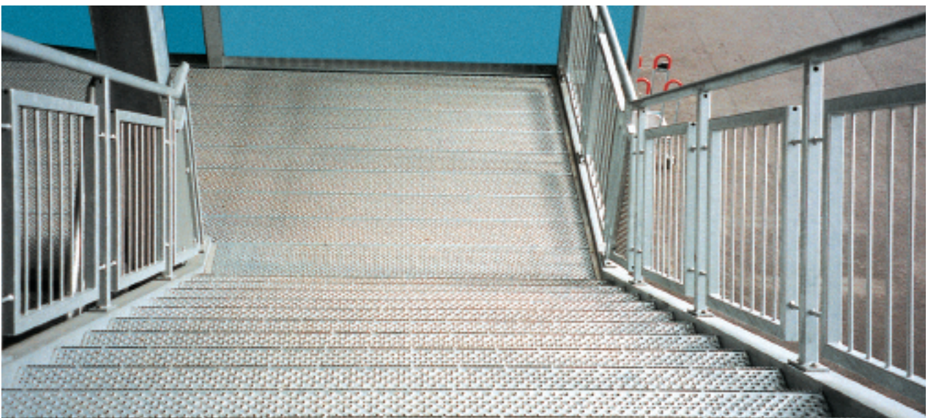
Staircase with intermediate landing
